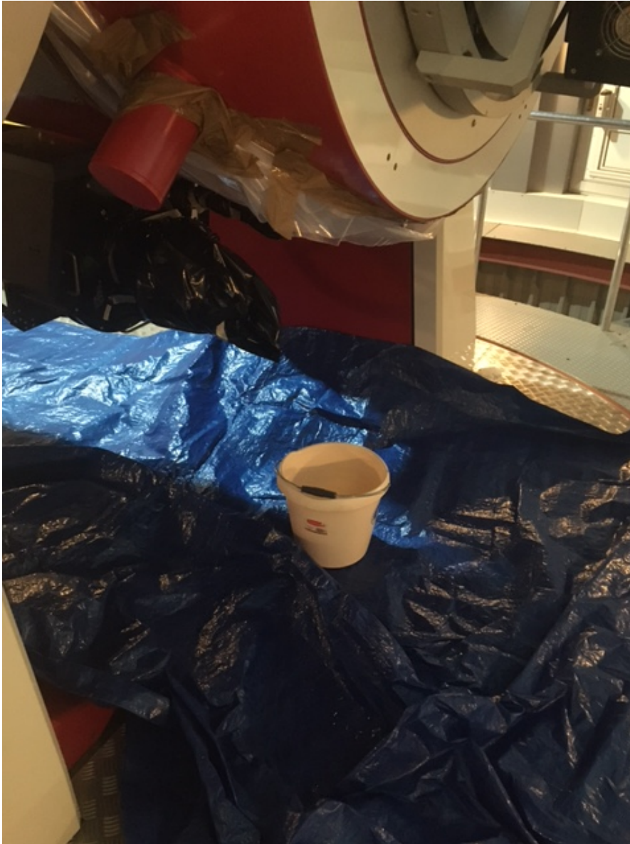
Fig. 7. Closing the lower half of the space between M1 cell and the tube in an attempt to control the direction of the water flow from M1 washing...and to avoid having water inside M1 cell.
