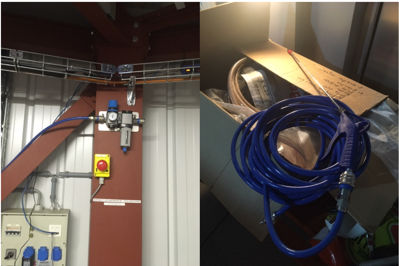
Fig. 2. Left hand panel: compressed air intake and filter, located just below the telescope floor; the pipe needs to be connected on the right hand side.
